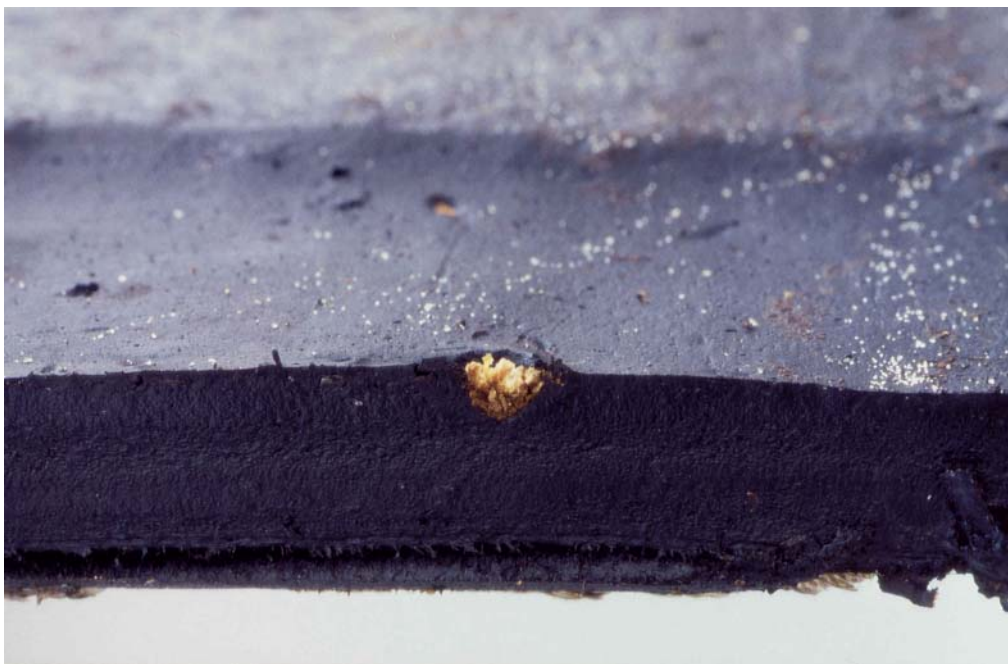
Figure 2: Cut through the sheet with root penetration
