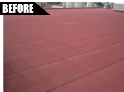
EXISTING ROOF WITH MINERAL WATERPROOFING MEMBRANE
