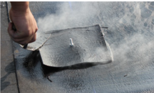
INSTALLATION OF THE SCREW FOR THE FIXING OF THE ELECTRICAL CONDUIT BRACKET WITH TORCH ON APPLICATION.
