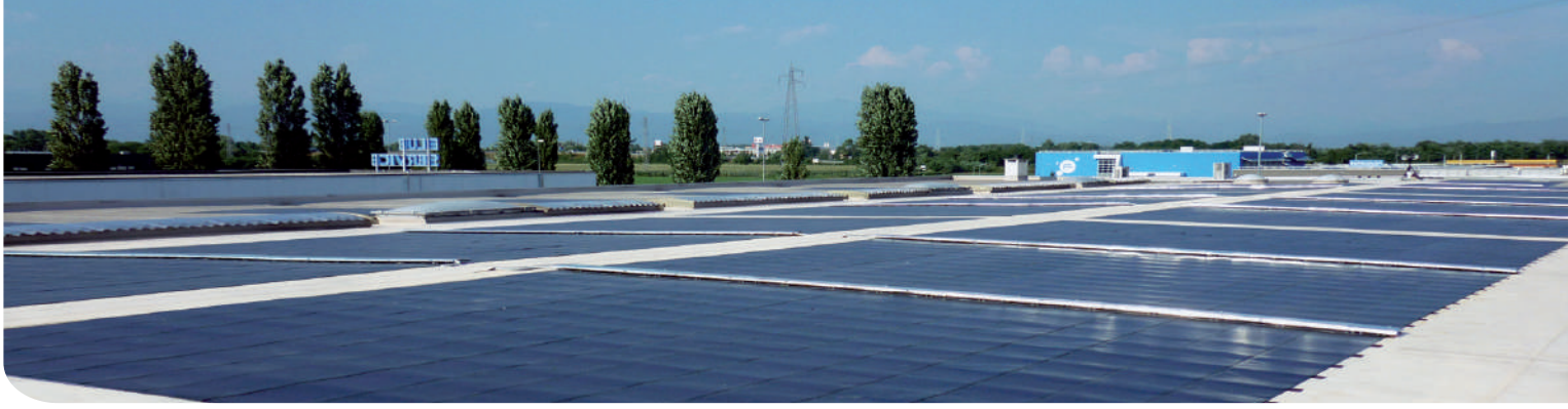
Fig. 3 General Solar PV on single ply Membrane Area: 3.500 m 2 - Power: 50 kWp
