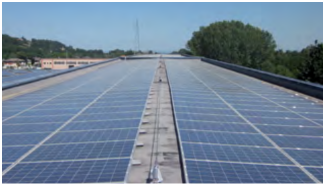
Photovoltaic modules fixed onto coverings waterproofed using the existing bituminous membranes and the General Fix EVO system.
