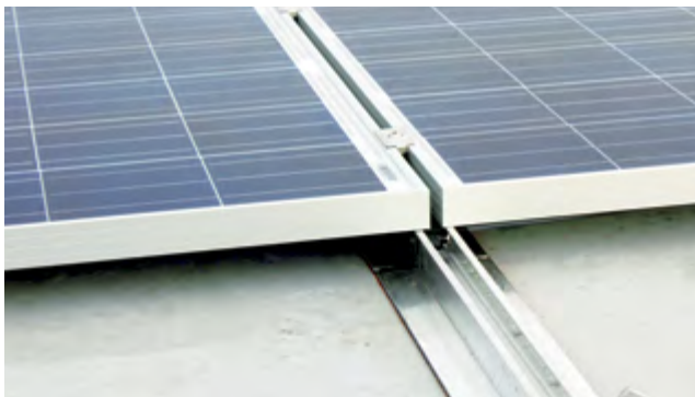
Photovoltaic modules fixed onto coverings waterproofed using the existing synthetic membranes and the General Fix system.
